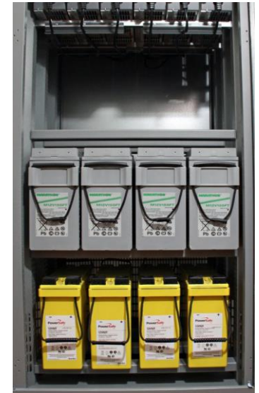
System measurements, diagnostics and parameter setting
